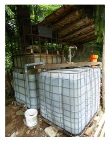
Building a simple Bio-Gas Plant (IBC System), with Shanti. Following instructions by Martin Funk right: fermenter in IBC tank (used) with filler neck (orange), gas tap (hose connection) and distributor, as well as overflow for fertilizer broth (left).
